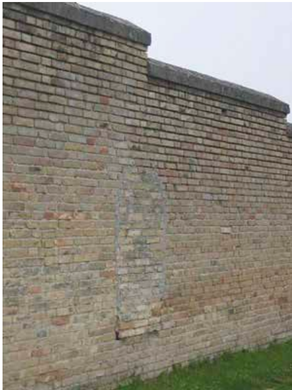
The hole in the wall (repaired) through which the POWs escaped.
